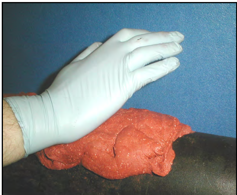
Figure 2-7: Applying DMP-3 Damping Material
