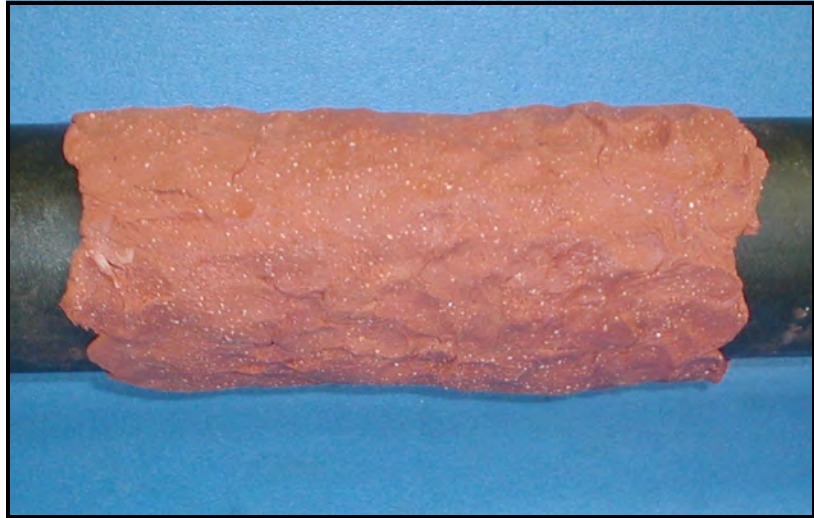
Figure 2-8: Spreading DMP-3 Damping Material
