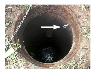
Figure 5: Eyebolt suspension in manhole
