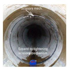
Figure 25: Expand and secure the ring against the channel wall
