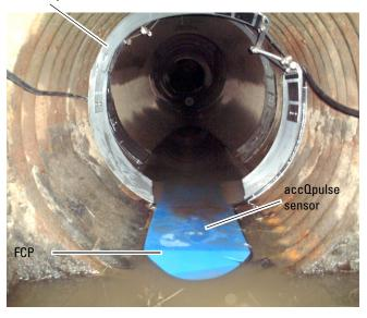
Figure 14: FCP and Scissors ring installation
