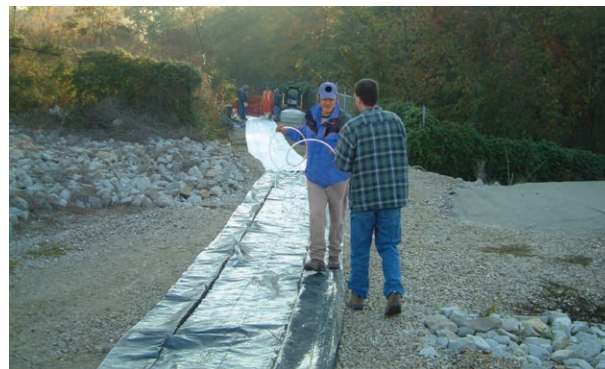
Figure 6-2 Tubing Being Pulled to Reference Mark
