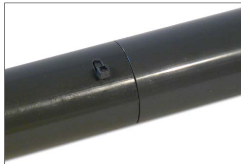
Figure 5-6 Cut Off the Excess Shear Tie
