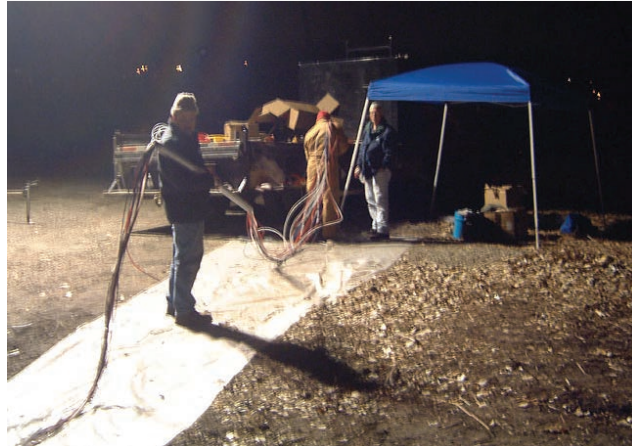
Figure 4-5 Casing Section Being Threaded Over Monitoring Tubing
