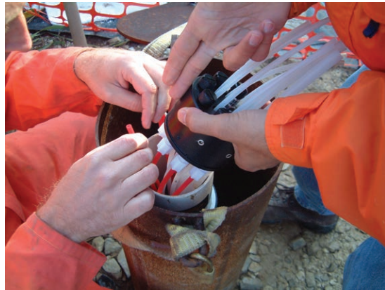
Figure 9-3 Pump Tubing Being Attached to a Wellhead
