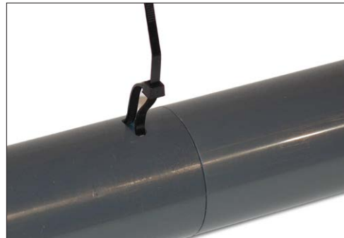
Figure 5-5 Pull Shear Tie Tight
