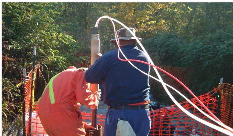
Figure 4-4 Initial Section Being Installed Down-hole
