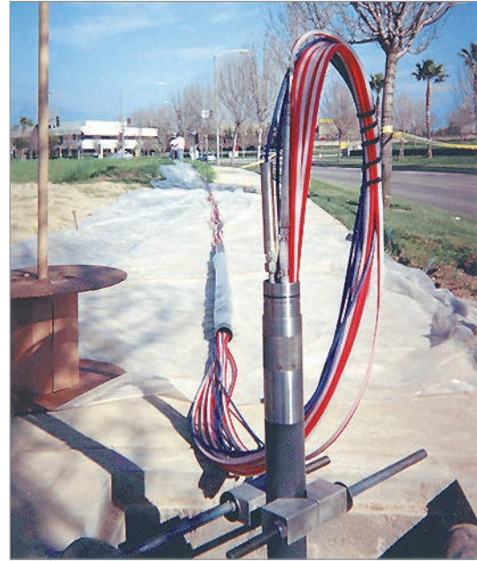
Contaminant investigation at a U.S. Air Force Base. Waterloo Systems installed to 213 m (700 ft) in overburden using screened and cased wells. Up to 6 zones per hole with dedicated pumps and transducers.
