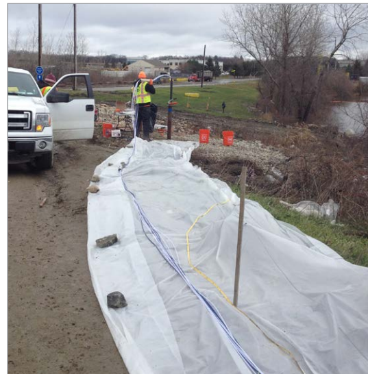
Five Waterloo Systems were installed to 33.5 m (110 ft) in fractured bedrock to help characterize a historical chlorobenzene plume at the site of a proposed groundwater pump and treat site. Vibrating Wire Transducers and Double Valve Pumps were dedicated at each of the 4 monitoring zones.
