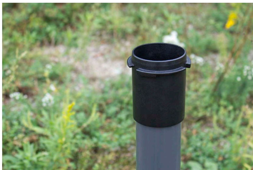
Figure 6-3 Install the Well Cap Base
