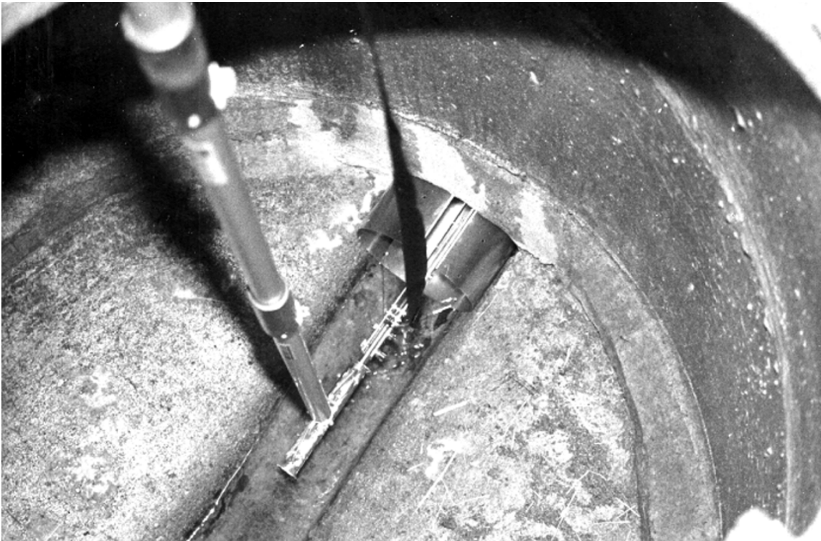
Figure 1-6 Inserting ring into upstream channel
